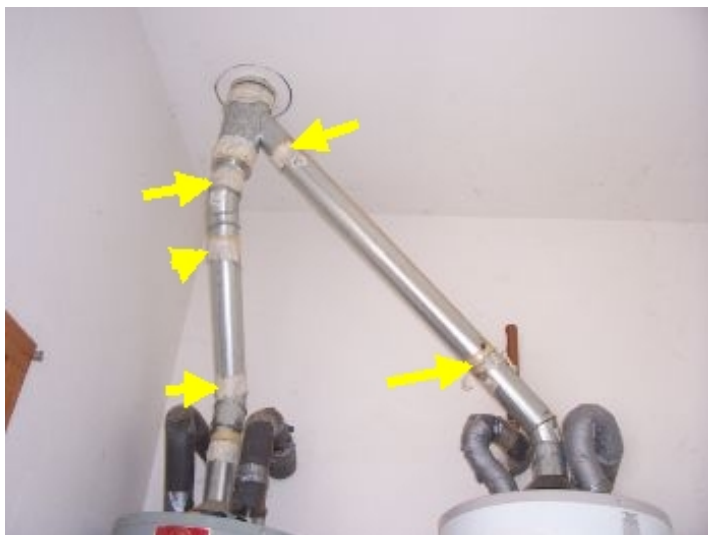
wrong type of tape on vent pipes
