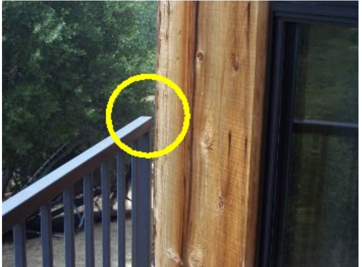
handrail is loose at wall
