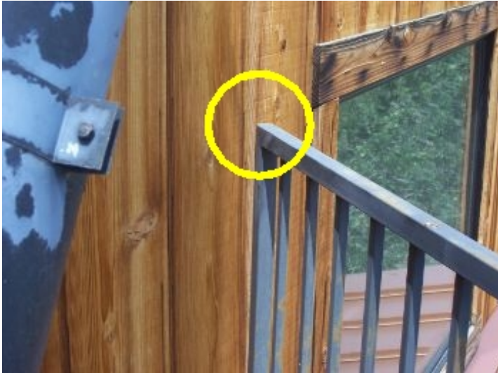
handrail is loose at wall
