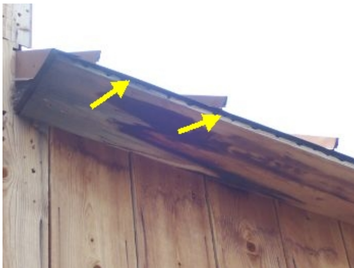
missing drip metal
