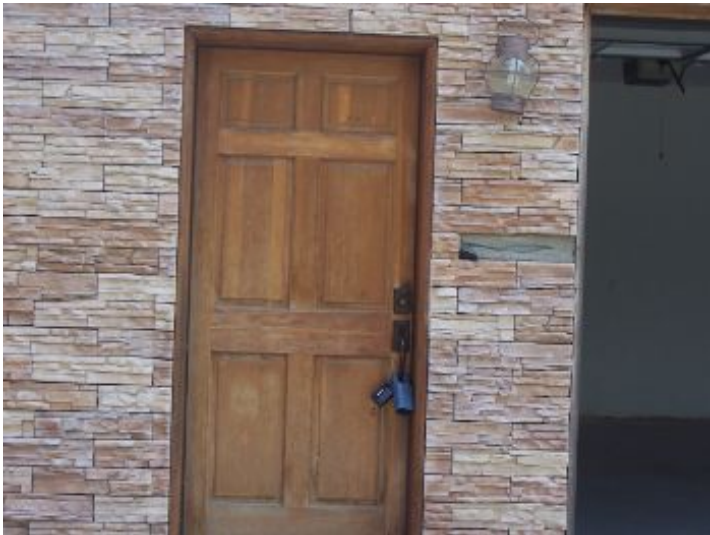
garage man door needs to be varnished
