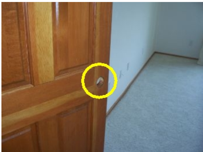
Bedroom #2 is missing door knob and striker plate on utility door.
