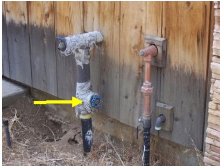
main water shut off at house
