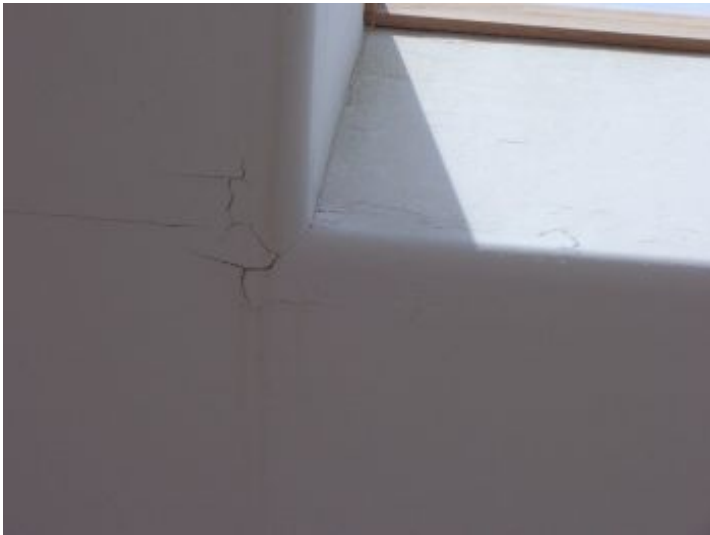
Master Bedroom loft ceiling at sky lights appear to have a leak.
