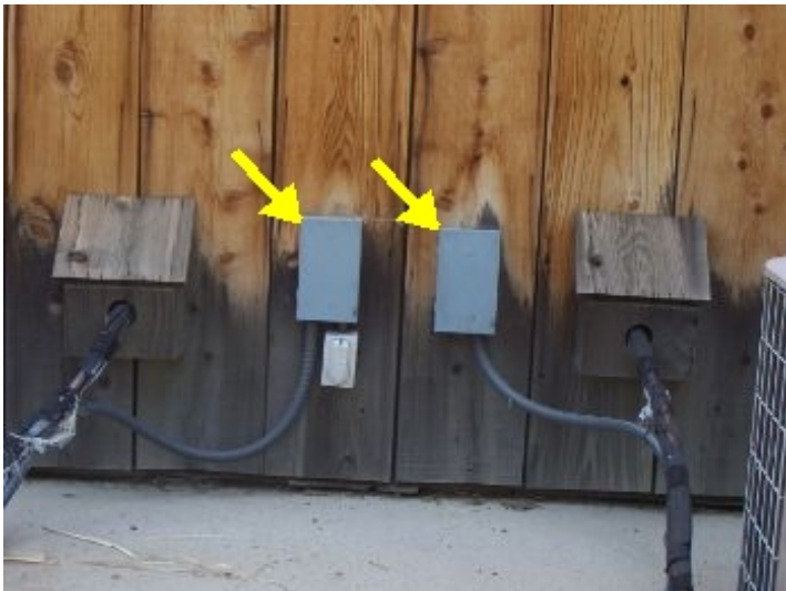
power disconnects for AC condensers
