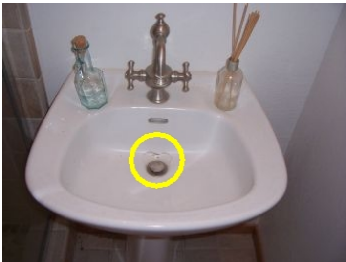
Sink is cracked around stopper area.
