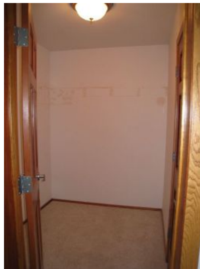
master closet missing shelf and pole
