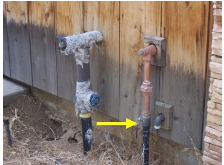
main gas shut off at house
