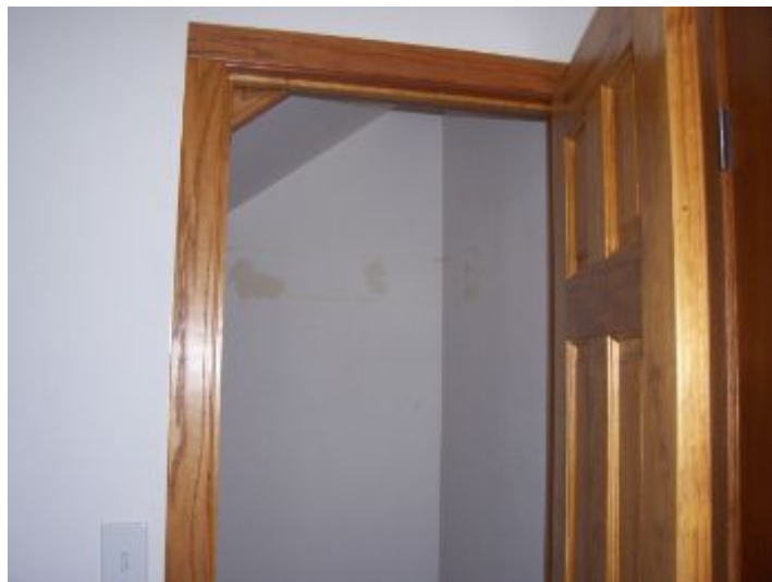
entry closet missing shelf and pole
